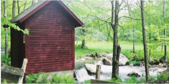
Figure 7. Furnace Brook Intake
