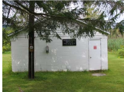
Figure 4. Field Street Well House
