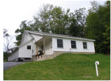
Figure 1. Proctor Filter Plant
