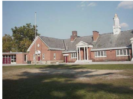
Proctor's attractive, brick-built, Elementary School underwent significant improvements in 2002.
