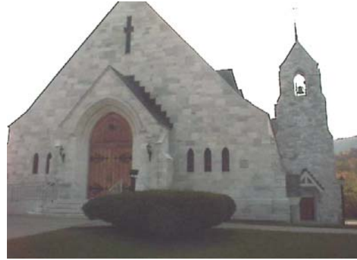
St Dominic's Roman Catholic Church, 1925, Neo-Gothic Revival. Built of local materials, the walls are faced with smooth blocks of marble and the roof is covered with many rows of longwearing slate.
